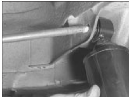
16.2a Removing a shock absorber upper mounting ...
