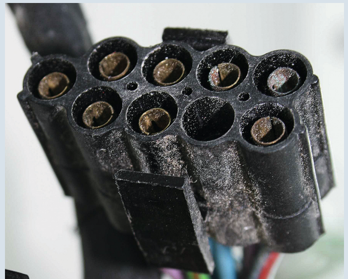
Figure 1: A common nuisance: Faulty electrical connections.
