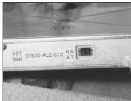
11.9 The ECU viewing window where the red and yellow LEDs can be seen (driver's seat removed for clarity)
