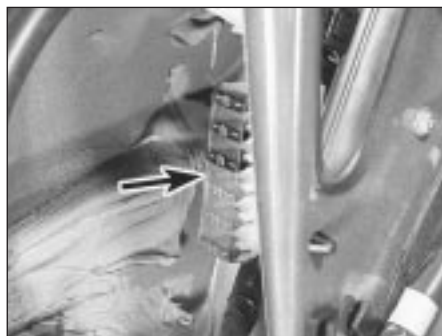
3.11 Luggage compartment fusebox (arrowed) located behind the left-hand side interior trim panel
