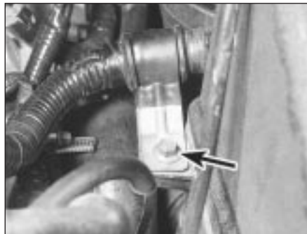
2.8b . . . and undo the wiring harness support clip bolt (arrowed) at the rear
